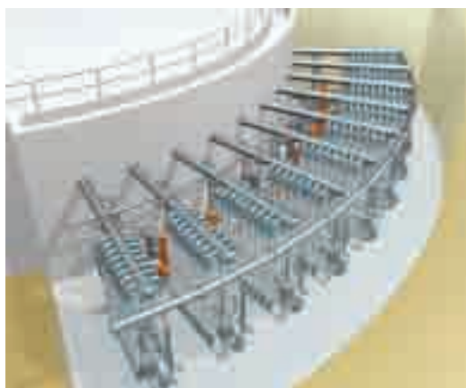
Membrane Skids positioned around BR Tank (under construction, Palm Is., Dubai. 17 MLD)
