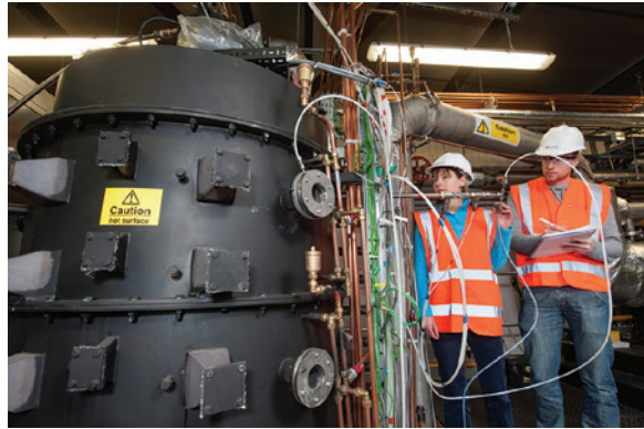
Upper section of the 250kW Air-Oxyfule combustion plant
