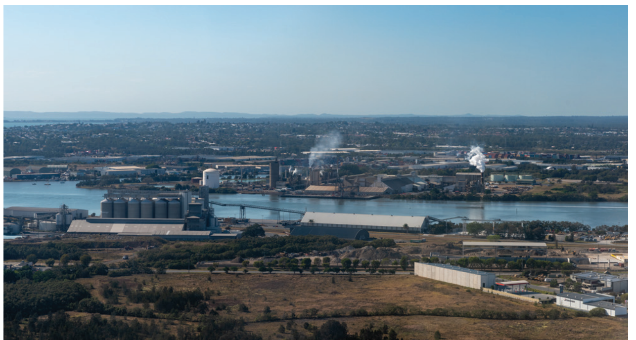
Gibson Island Ammonia, Urea and CO 2 Carbon Capture and purification plant, Brisbane Australia
