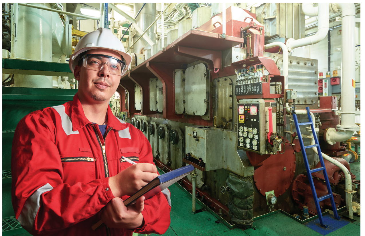
Ship's engine room
