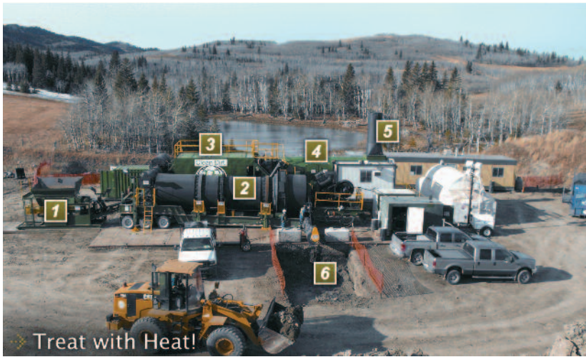
Fig 3. (a) & (b) Stages of the MTSR system (90,000 tonne soil remediation in Pincher Creek, Alberta, Canada)
