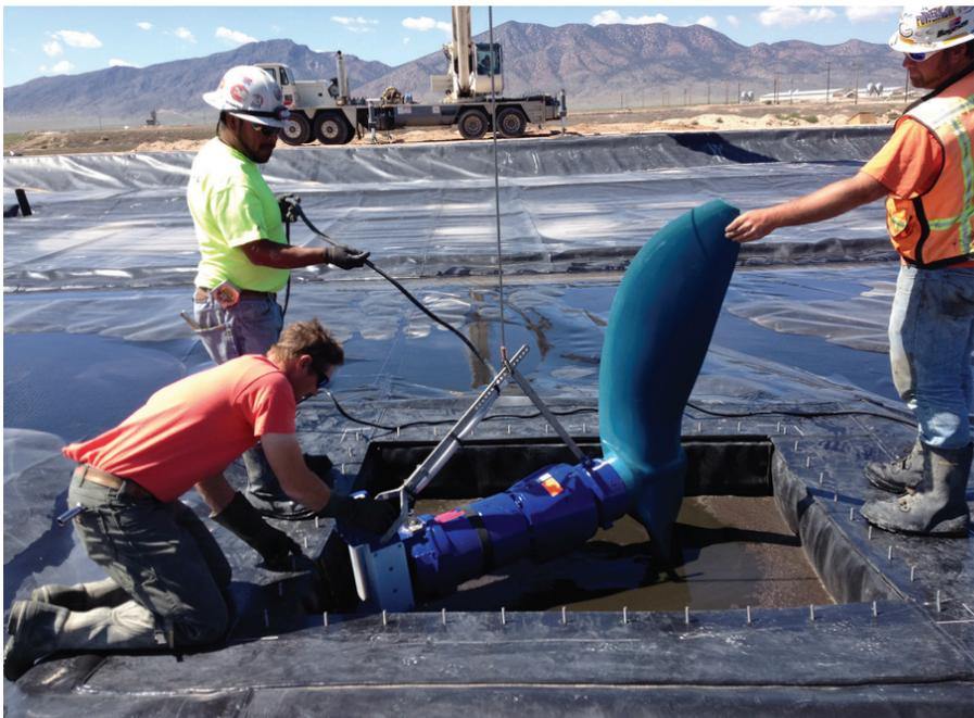
Fig.4. KSB Amaprop K42-2500/65ZEG mixer being installed in the 11 million gallon digester basin.
