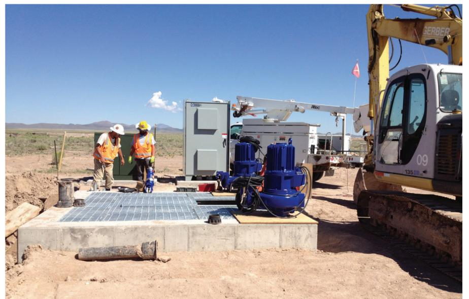
Fig.2. KSB Amarex KRT vertical submersible effluent pump.
