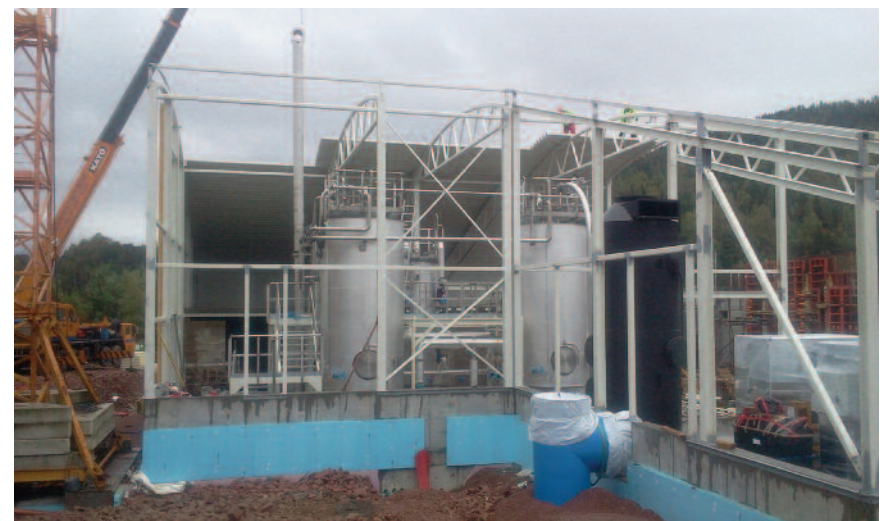
Figure 5: THP at Lindum under construction
