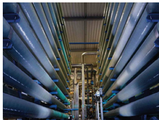
RO elements at Terneuzen treat 7,500 m 3 /day of challenging feed water (Photo courtesy of Evides Industriewater B.V.).
