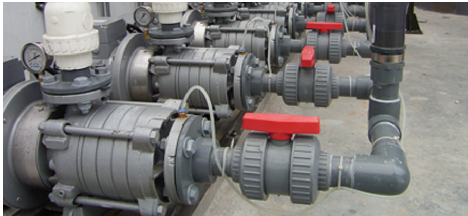
Figure 4: Innovative dissolved air flotation unit with EDUR multiphase pumps (illustration supplied by: MGCC)
