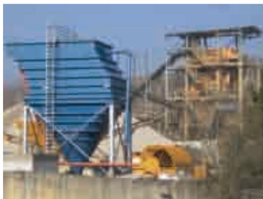
fig.1: installation of the treatment plant with Leiblein lamella separator
