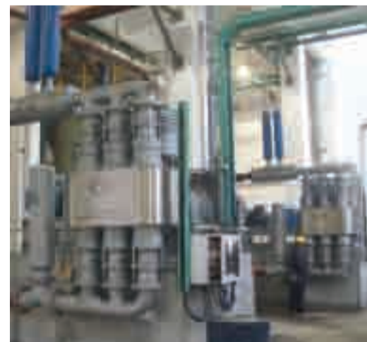
Fig. 2 Multisafe Pumps are available for max. flow rates of 600 m 3 /h (6 pump heads) and max. pressures of 320 bar
