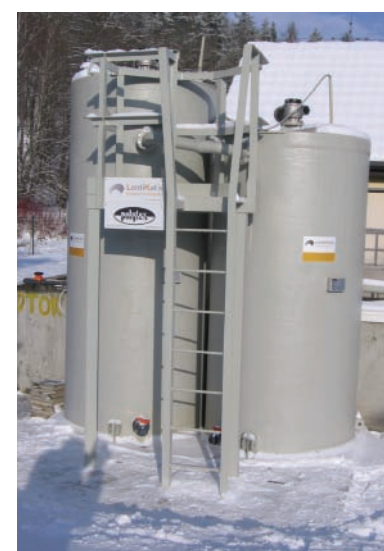
Figure 3: Full-scale application (WWTP Ostrov u Macochy, Czech Republic) – removal of residual nitrates.
