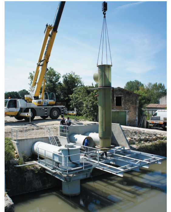
Fig. 2 Engineering work being undertaken at Sylvéreal.
