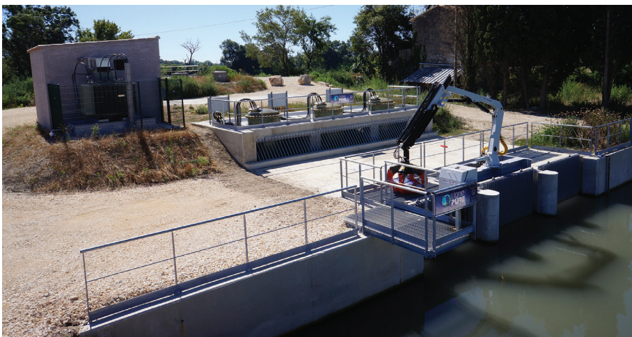
Fig.1 The new pumping station at La Capette.
