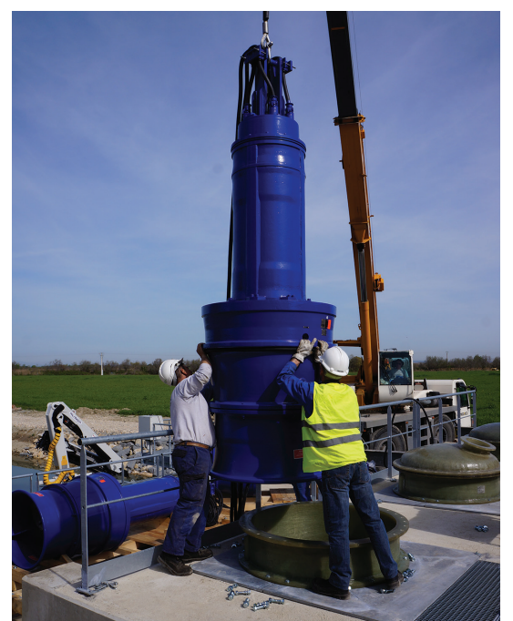
Fig. 3 The Amacan P is a close-coupled wet installed single entry axial open impeller pump.
