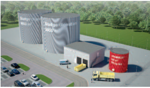
Process layout for application of ANAMMOX® as water post-treatment of sludge digestion
