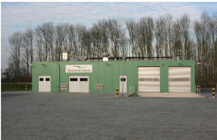
Waste water treatment plant at Aviko Steenderen
