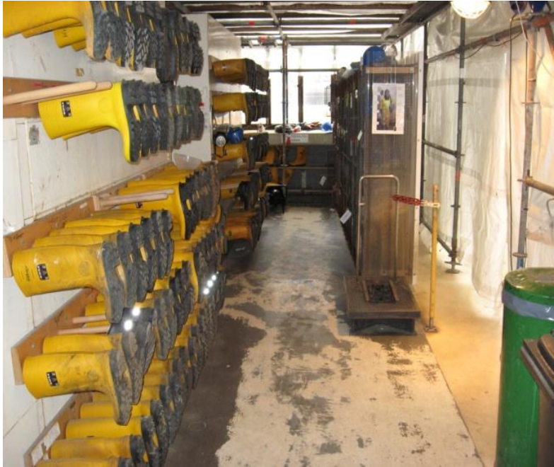
Installation of dedicated area to change PPE: Personal protective equipment
